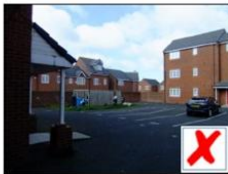
Example of poor provision of communal bin store facility which is remote from residents and no access for collection vehicles.
