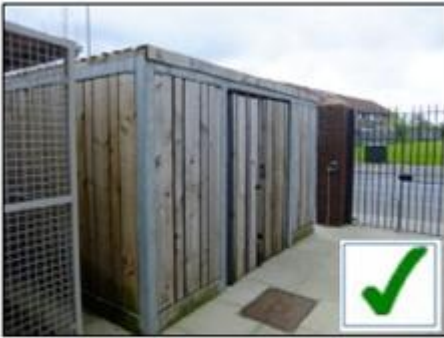
Good example secure communal bin store provision. Store is easily accessed by residents, is ventilated and aesthetically appealing with access for waste collection crews to collect bins.
