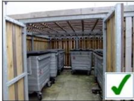
Good example of secure communal bin store, where inside is ventilated with a drain for cleaning.
