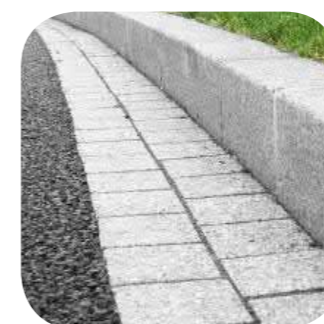
Kerb & Block Paving Channel
