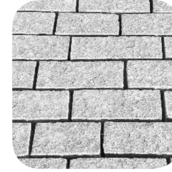
4 Block Paving (On carriageway)
