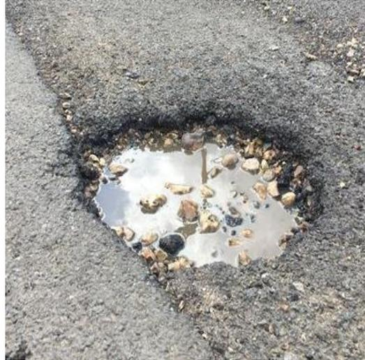
Water penetrates through cracks in the road surface and freezes when temperatures drop. The expansion and contraction process when water freezes and thaws undermines the stability of the road surface, causing damage to the surface.
