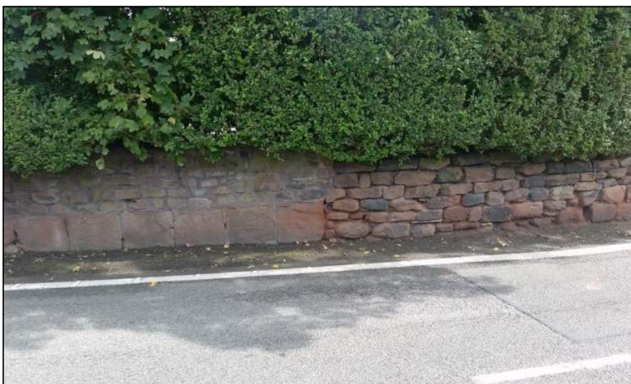
Figure 6 – An example of a remaining property boundary wall at Hall Lane, that is maintained to a good standard.
