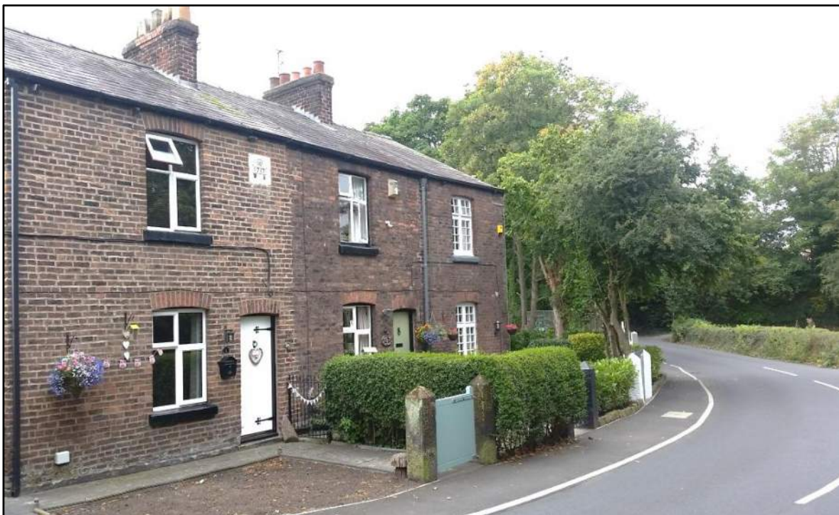
Figure 16 –Town End Cottages, date from the 19 th century of brick laid in common bond.
