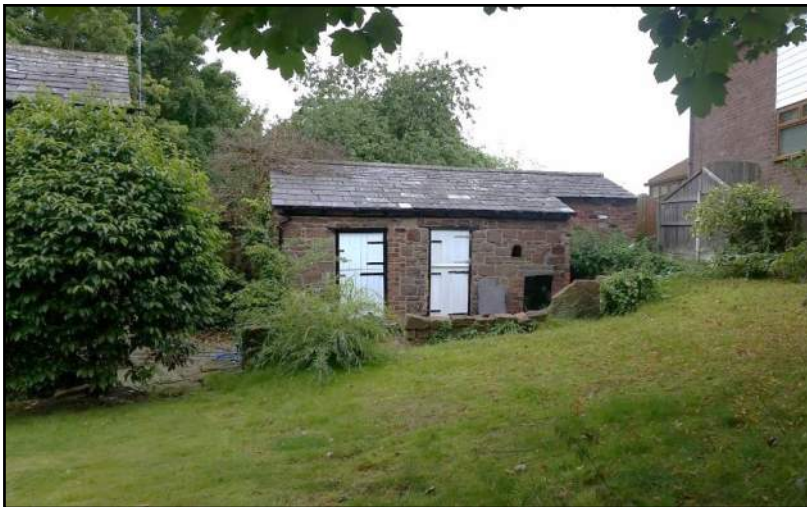
Figure 14 – Outbuildings at Sunnyside Farm, built using sandstone, likely to be from the former quarry on Pex Hill.
