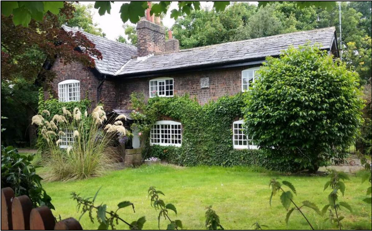
Figure 12 – Typical early horizontal sliding sash windows with small panes, few original windows remain within the conservation area with many significantly altered.
