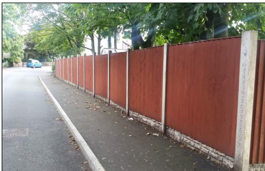
Figure 7 – Tall wooden fencing creates an imposing inactive frontage that detracts from the wider natural setting of the conservation area at Hall Lane.
