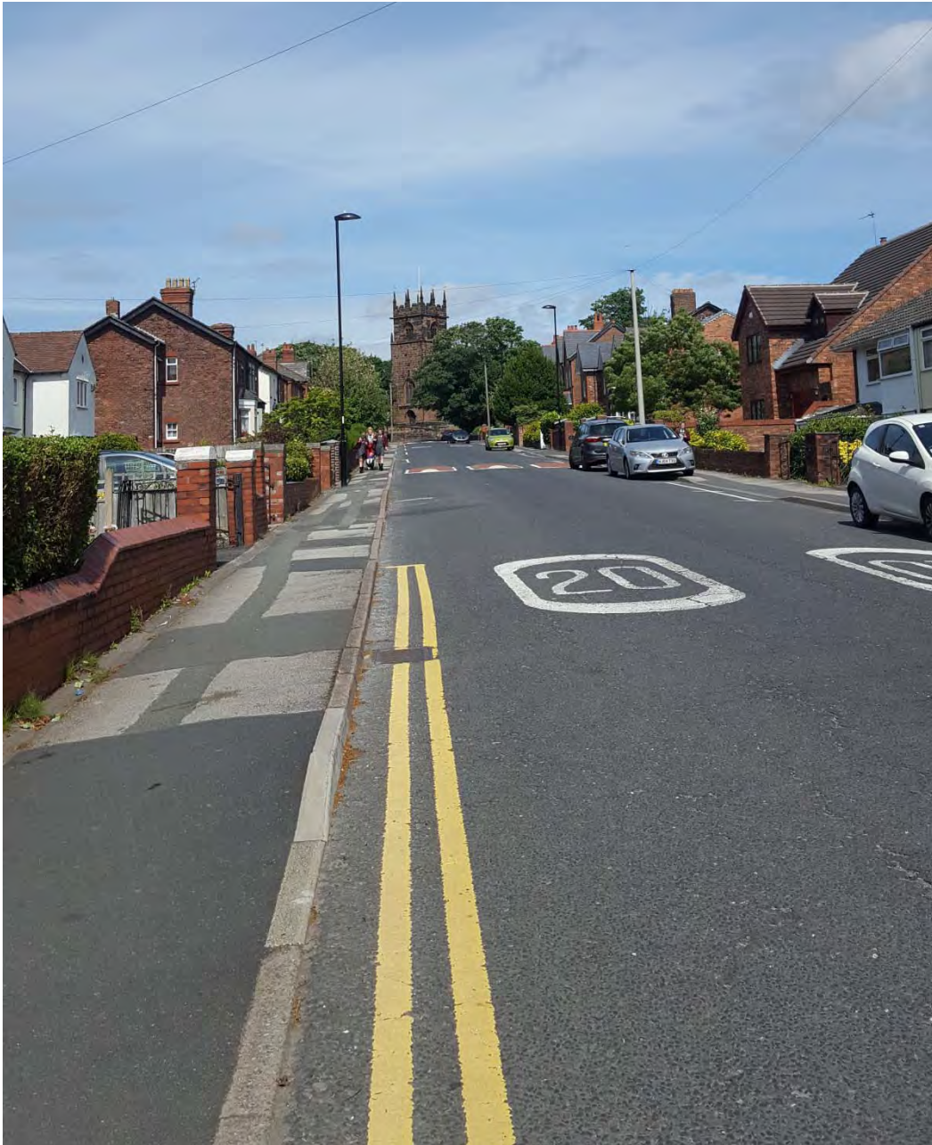
Figure 11 - This view along Stanley Road shows the prominence of the church, but also the negative impact the road markings and speed cushions have on the appearance of the area.
