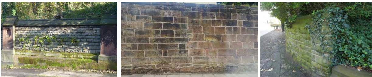
Figure 18 – Distinctive sandstone walls add to the character of the area.
