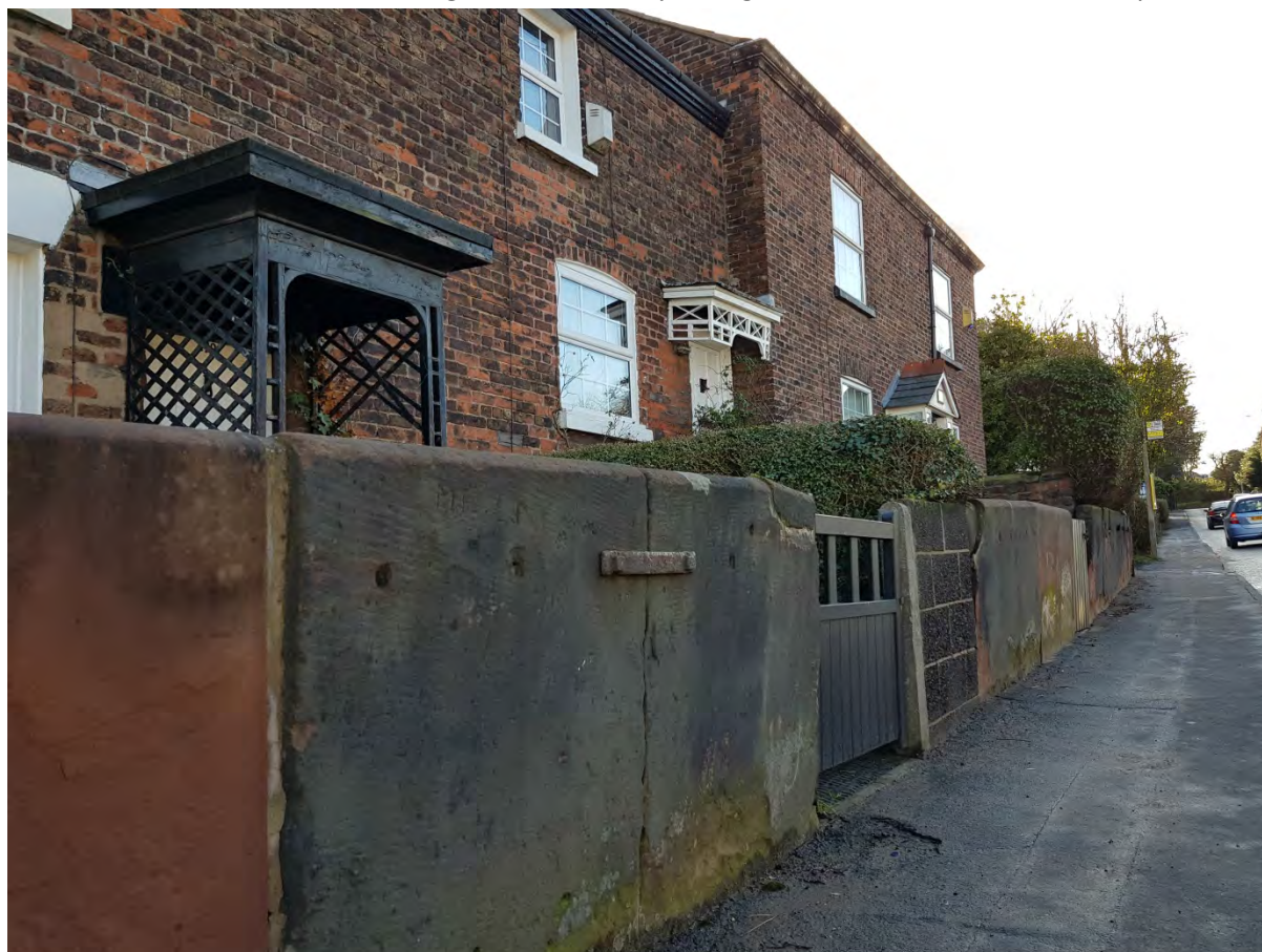
Figure 19 - Blue Bell Lane Showing Stone-Slab Walls with Modern Insertions and Irregular Plot Sizes and Building Lines of this Early Terrace.
