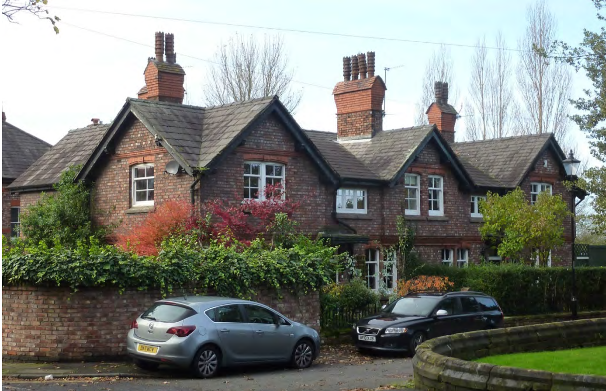
Figure 16 - Nos 1-3 Stanley Road, Showing Distinctive Chimneys, Brickwork and Prominent Gables
