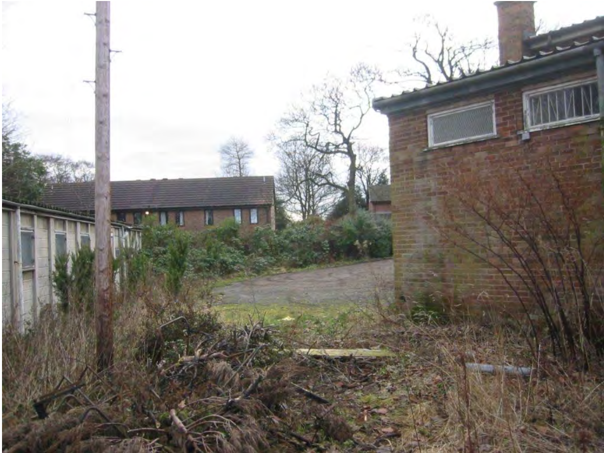
Figure 17 - Land north of St. Michael's Church Showing 20 th Century Buildings and the Houses in Capper Grove
