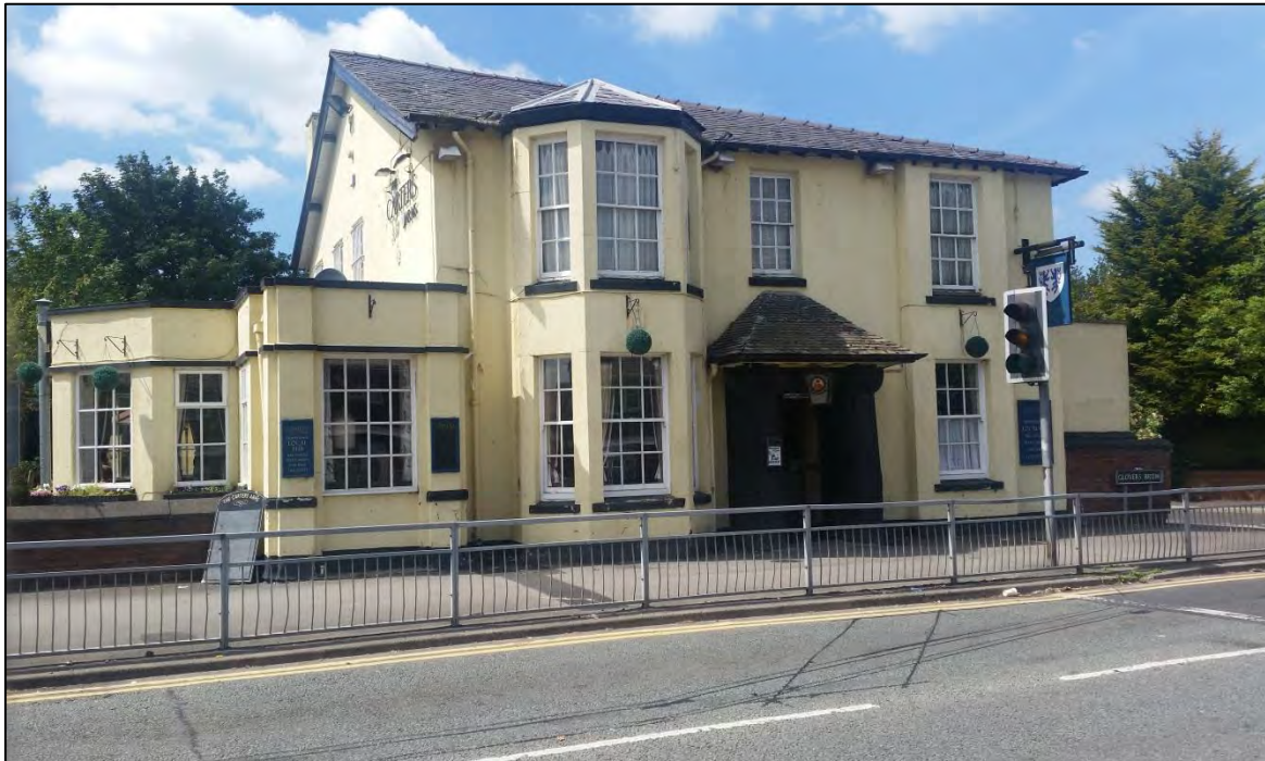
Figure 8 – The Carter’s Arms Public House is a focal building on Glover’s Brow located at the eastern entrance to North Park Road Conservation Area.
