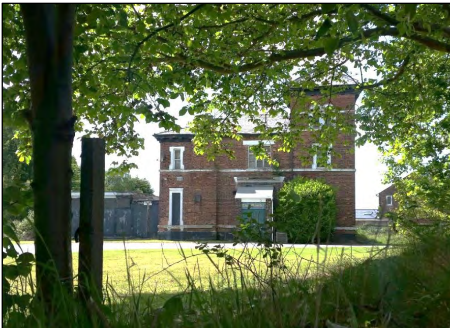
Figure 7 – The former Conservative Club on South Park Road known as Waverley House, dates to the 1800s and is a Grade II listed building. The site is in occasional use as Kirkby Conservative Club but has been subject to neglect, in addition to some earlier poor quality extensions that detract from the building.
