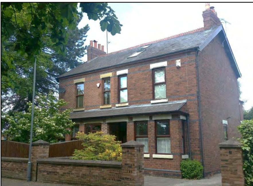
Figure 8 – 30 & 32 North Park Road, built in the 1900s display a good example of the smaller scale late Victorian development, with stone headers and sills to the windows.
