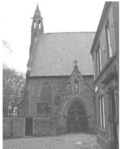
Date of Photograph: 1998. The Roman Catholic Church of 'Our Lady of the Immaculate Conception and St. Joseph', is located at the end of Vicarage Place, Prescot. It was built in 1856 by J. A. Hansom, the inventor of the Hansom 'cab.' Vicarage Place appears to have changed very little since the mid-nineteenth century and although restoration work has been carried out in this area, it has been completed sympathetically to its surroundings.
