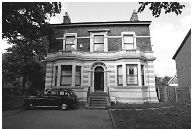
16 North Park Road. Victorian Brick House with stuccoed ground floor, arched doorway and fanlight.
